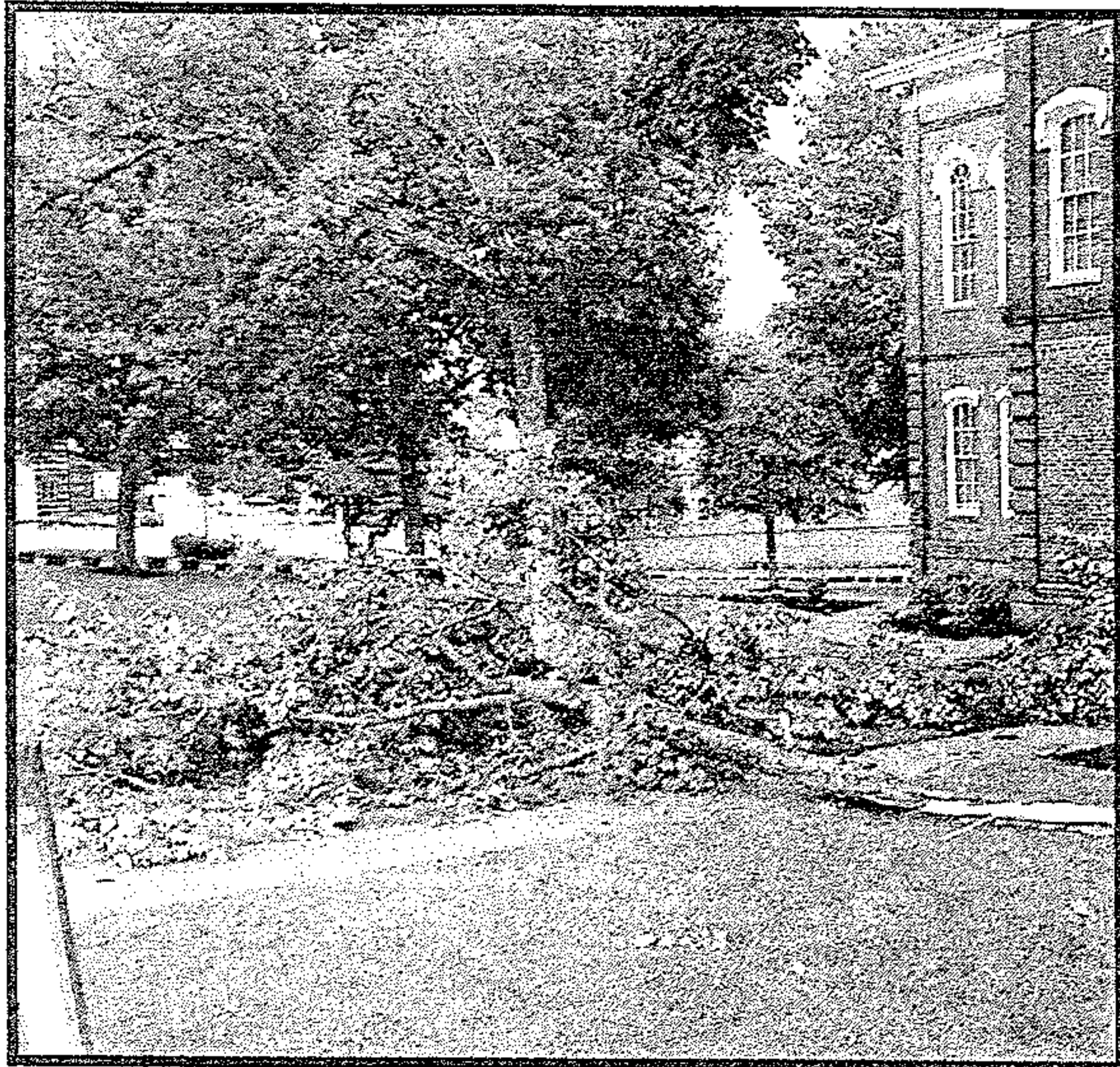
It's inevitable, if there is a storm the courthouse in Loudon WILL have some damage guaranteed. At least it didn't take out the roof this time.
